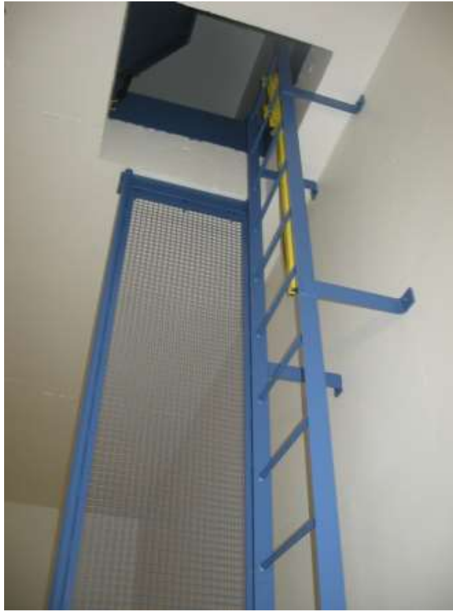
Finished / installed fall protection screen
