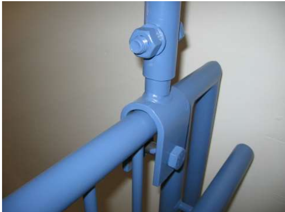
Finished / installed fall protection screen
